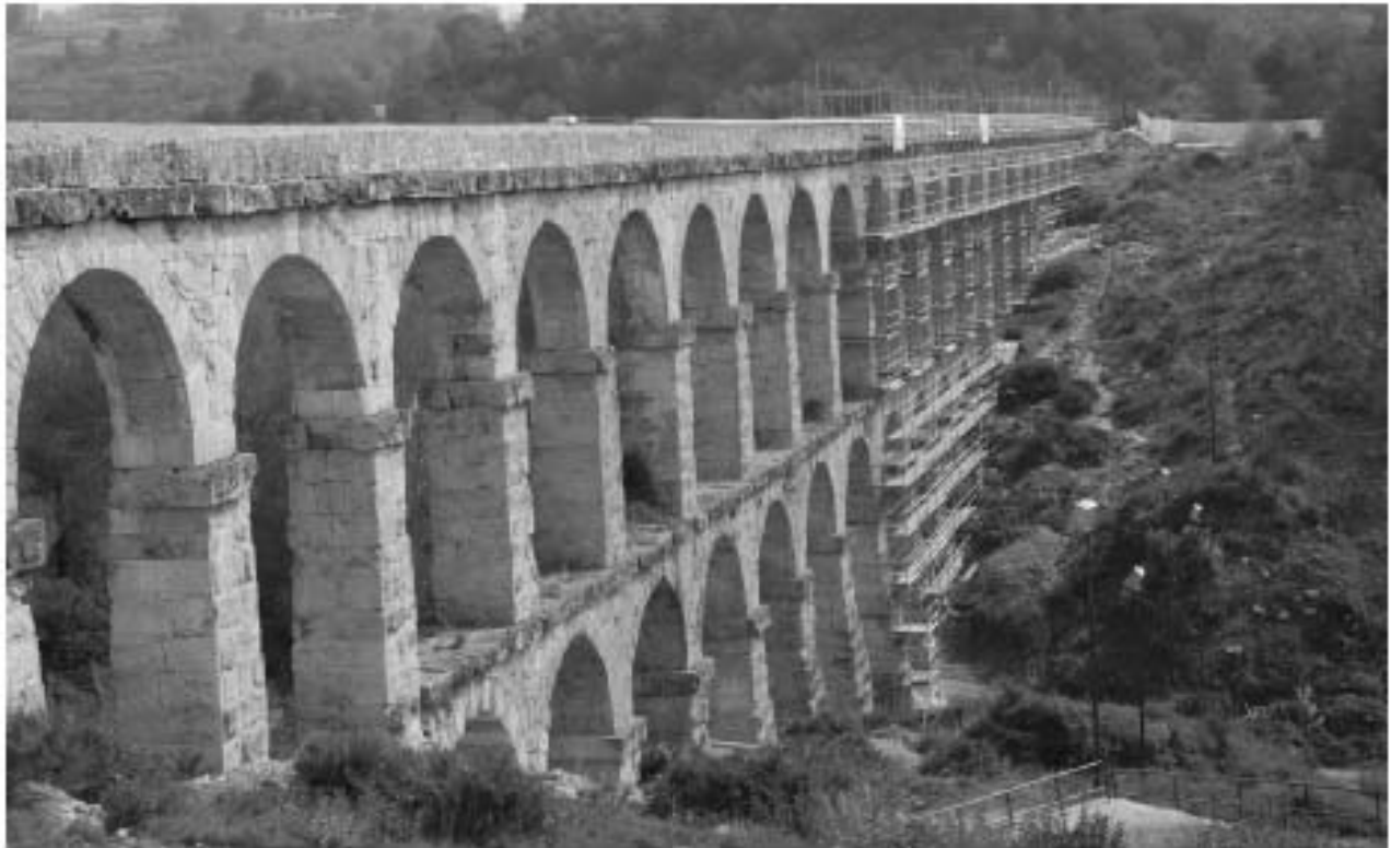
Fig. 10. Part of the aqueduct during its recent restoration.
