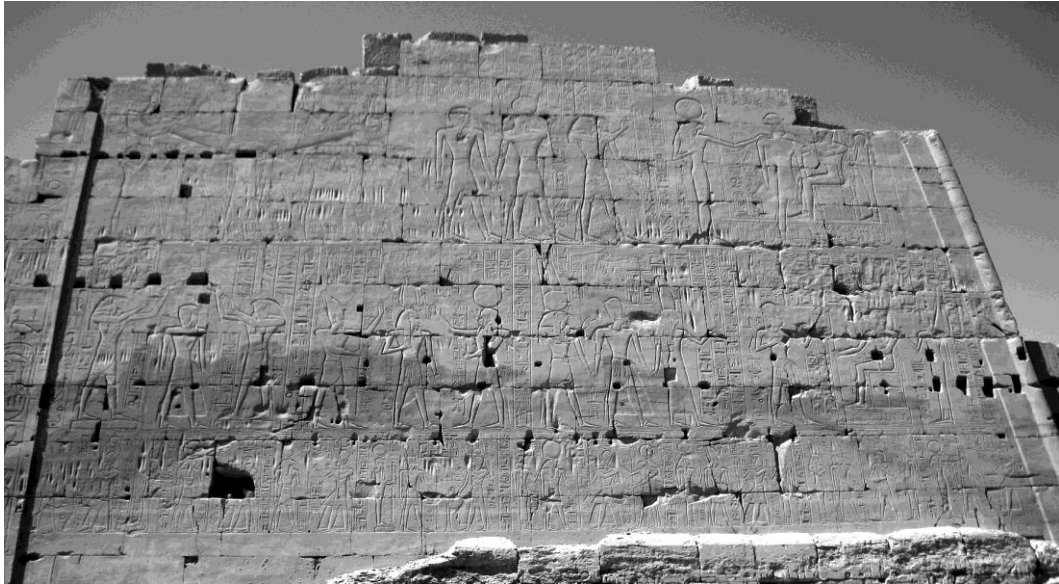
Figure 1: North face of the west tower of the eighth pylon at Karnak
