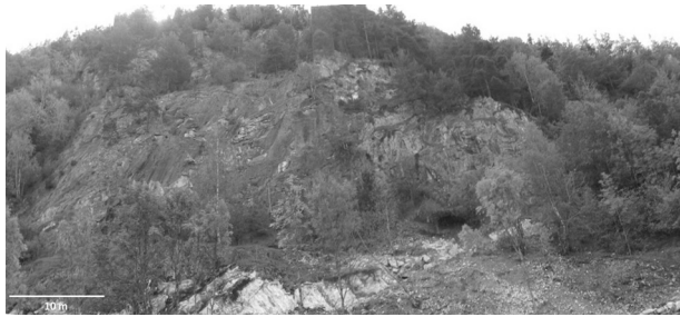
Fig. 3. View of Arties quarry front, seen from the north side. Samples were taken on the embankments of the actual access ramp located in the foreground.
