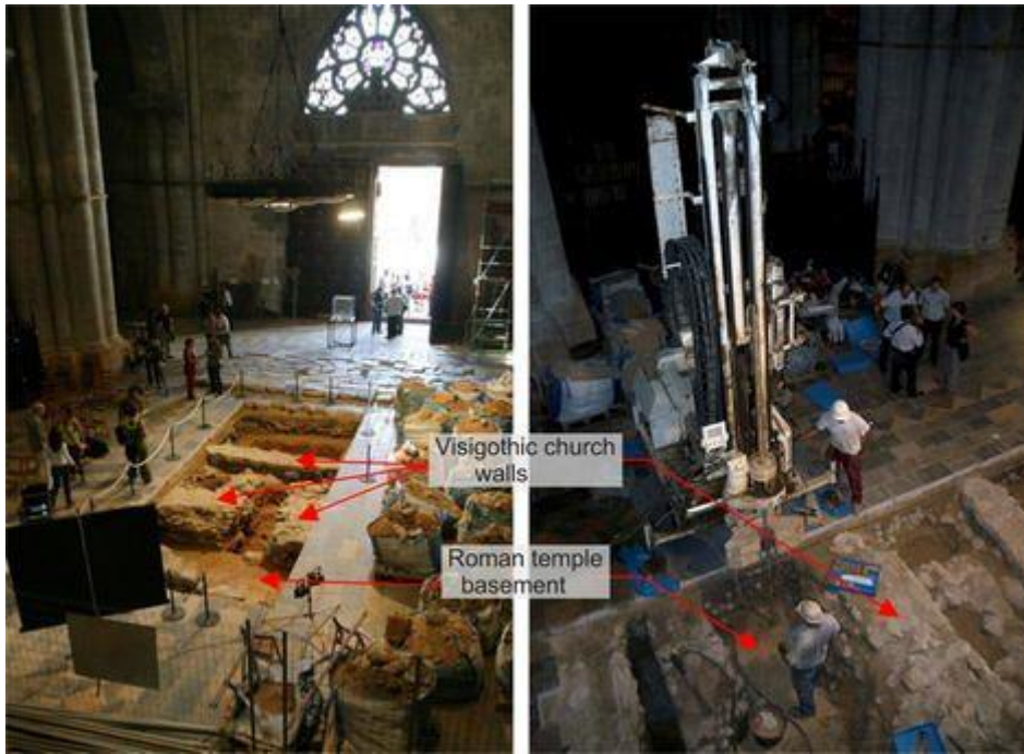
Figure 11. a Archaeological dig revealing the foundations of the Roman Temple and walls of Mediaeval buildings (left). b Borehole machine drilling inside the cathedral (right)
